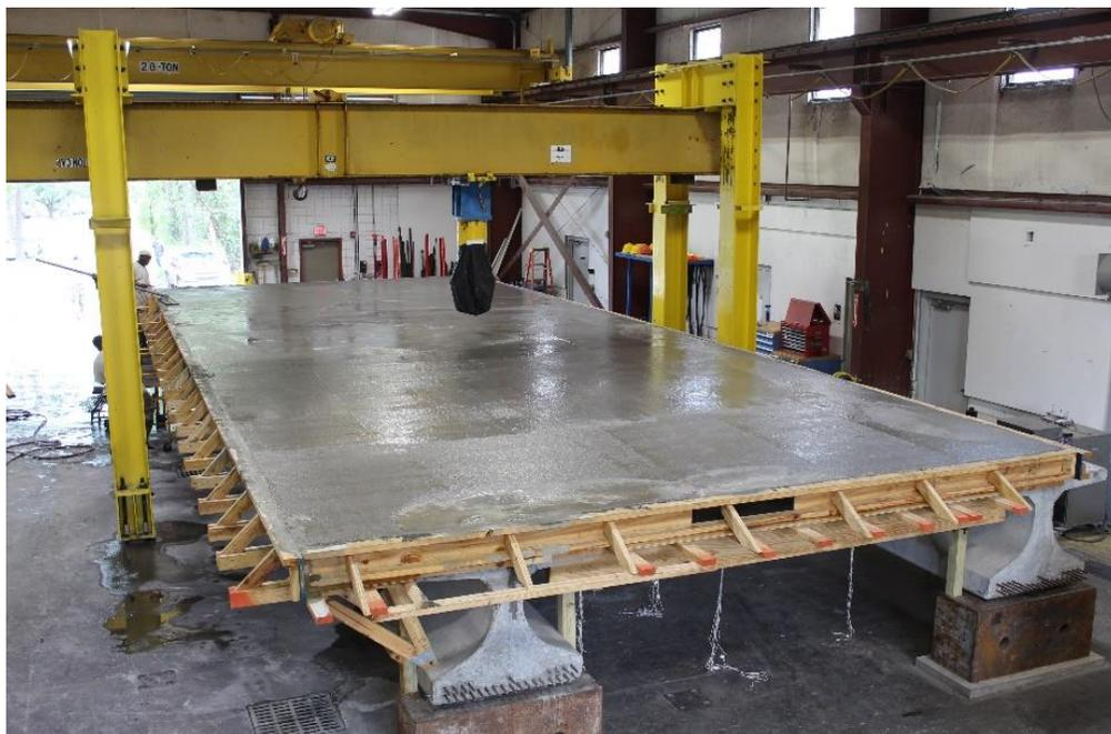
Figure 4.24: Concrete deck right after concrete pouring
