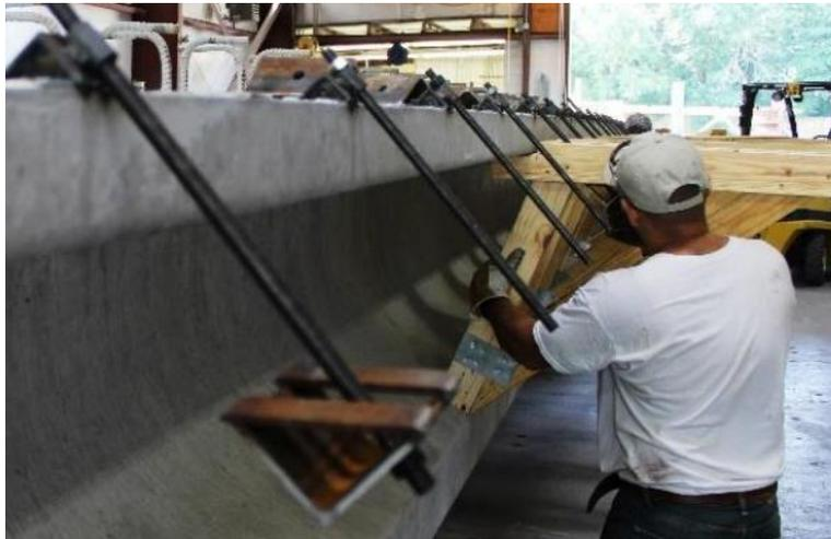
Figure 4.13: Adjusting cantilever formwork system
