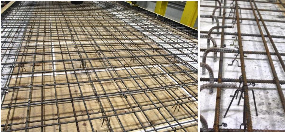
Figure 4.22: Placed top mat reinforcement
