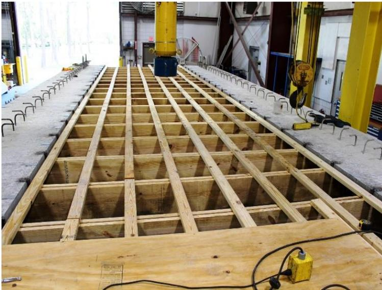
Figure 4.15: Deck formwork (clear span)
