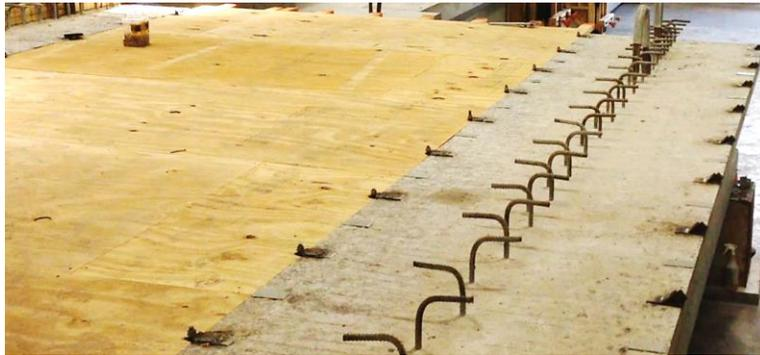
Figure 4.12: FIB-36 stirrups and overhang hanger brackets
