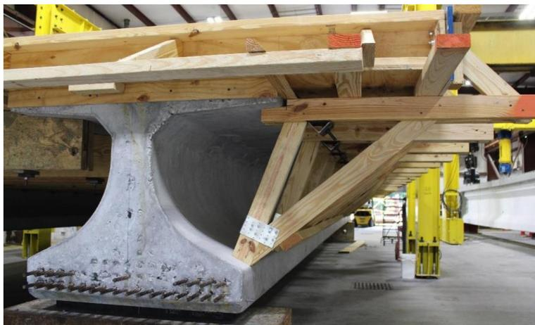
Figure 4.14: Cantilever formwork
