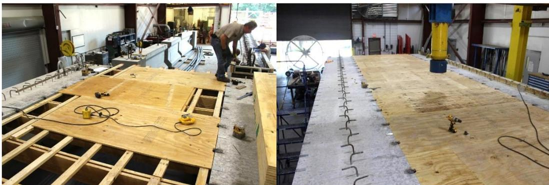
Figure 4.16: Deck formwork during construction
