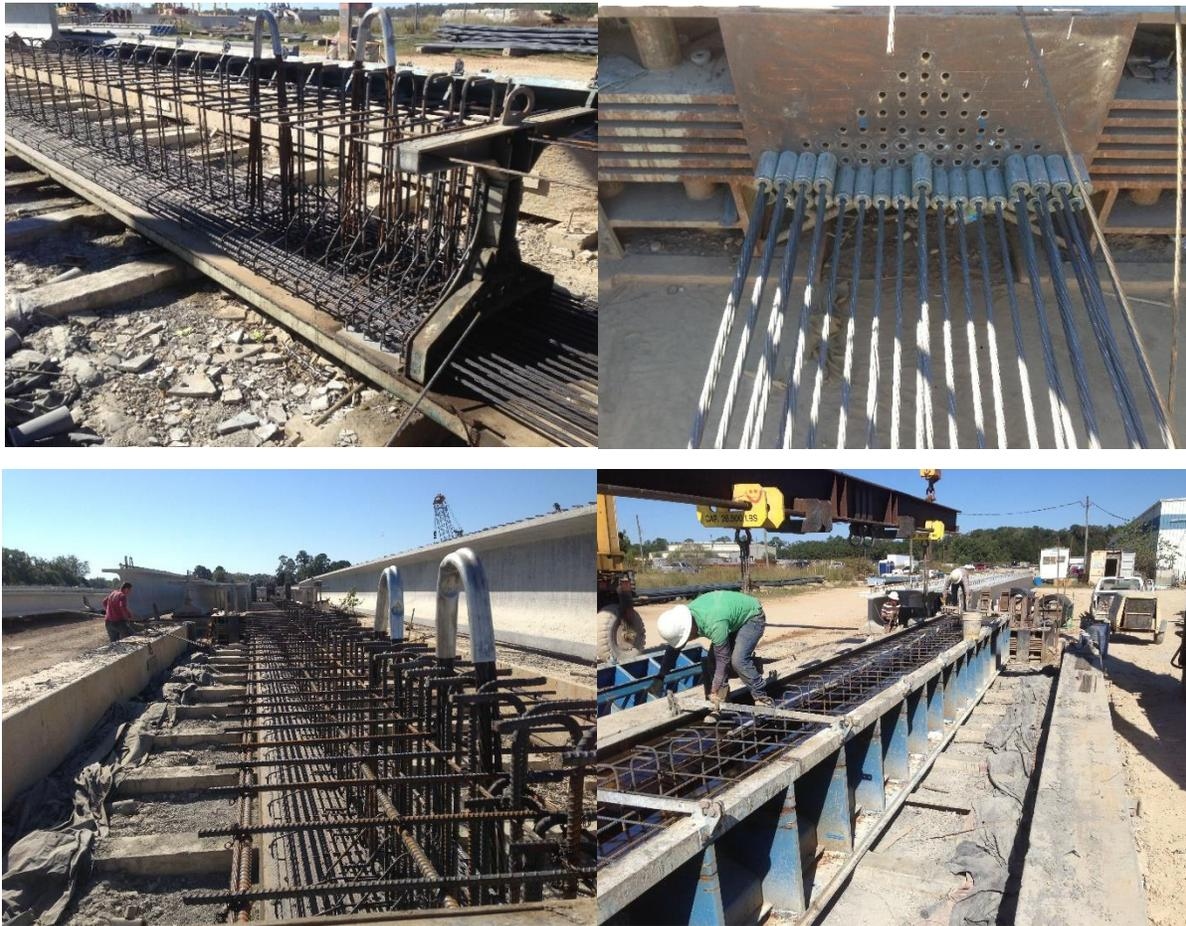
Figure 4.6: FIB-36 Fabrication showing formwork and prestressing tendons
