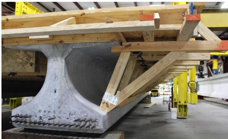
Figure 4.14: Cantilever formwork
